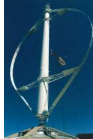
1985 Canada Darrieus 4MW, h=107m, d= 64m
