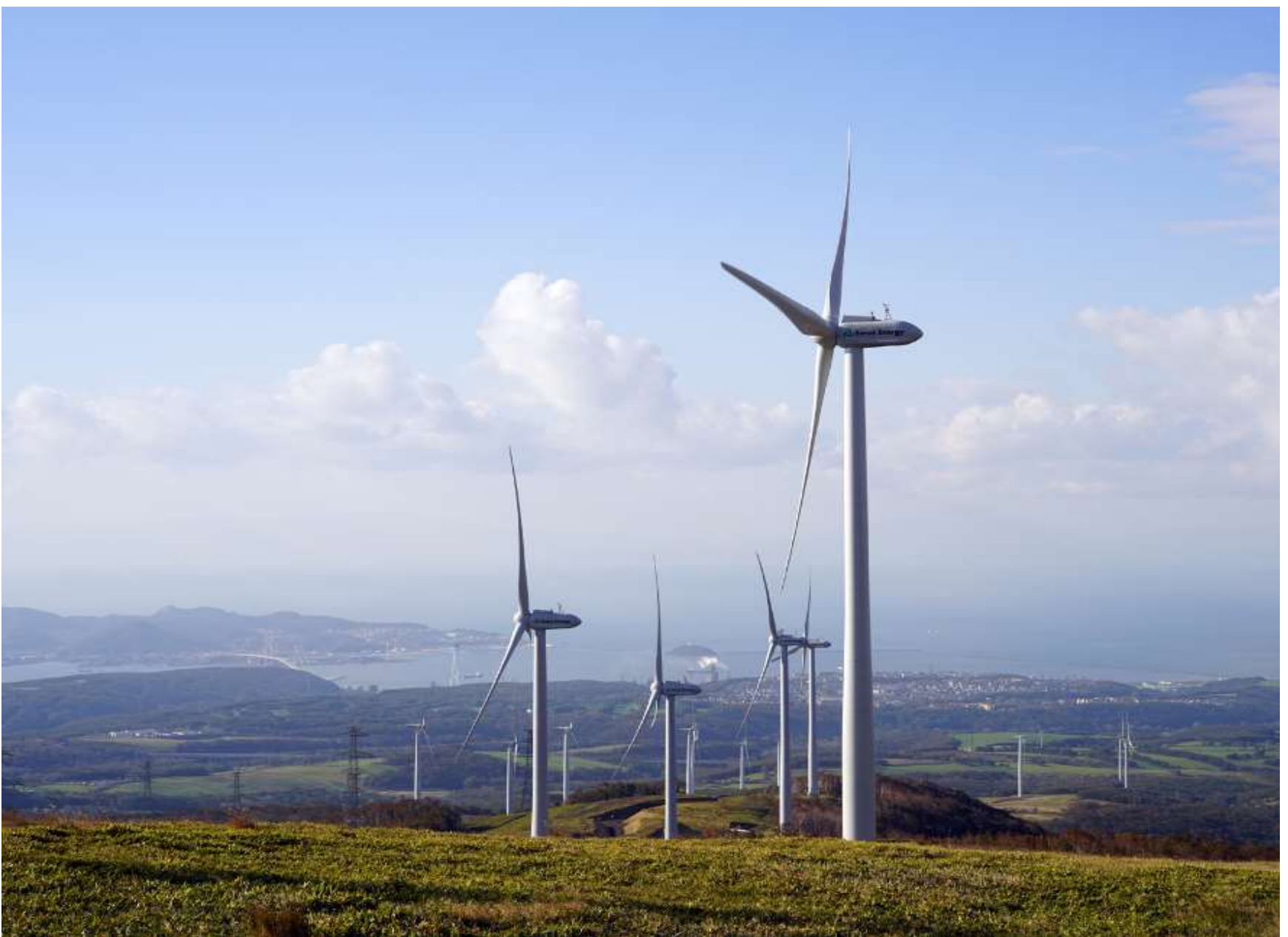
Typical Wind Farm in Japan; Hakodate in Hokkaido
