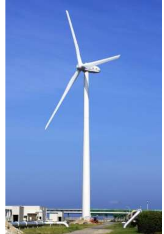
HITACHI 2.0 MW (5MW)
